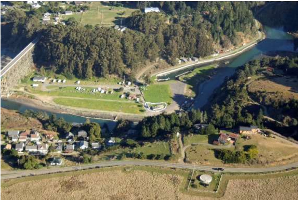
Figure 2-4: Albion and Schooner's Landing Marina
