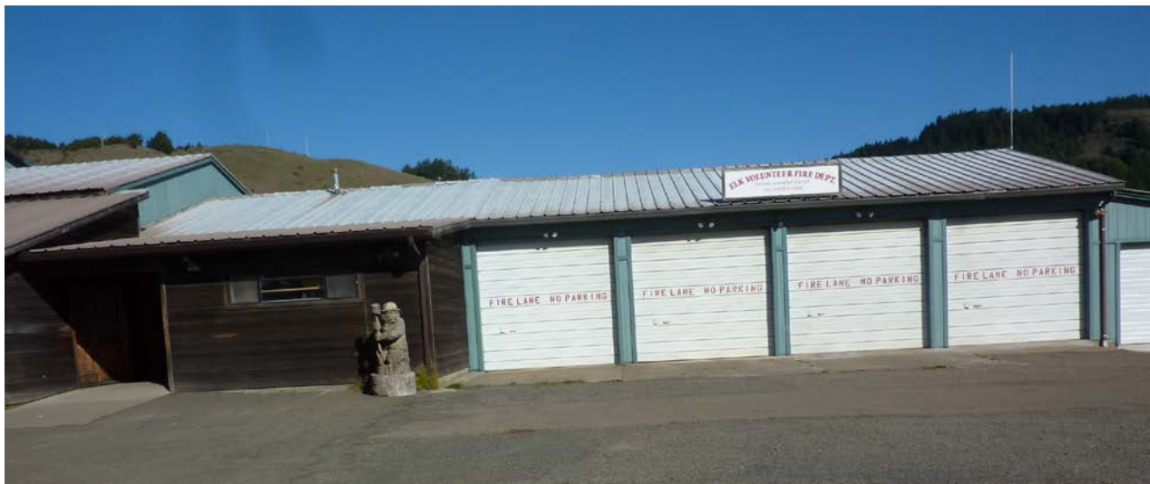
Main Fire Station The Skilton/McKnight Station 6129 S Highway 1 Elk
