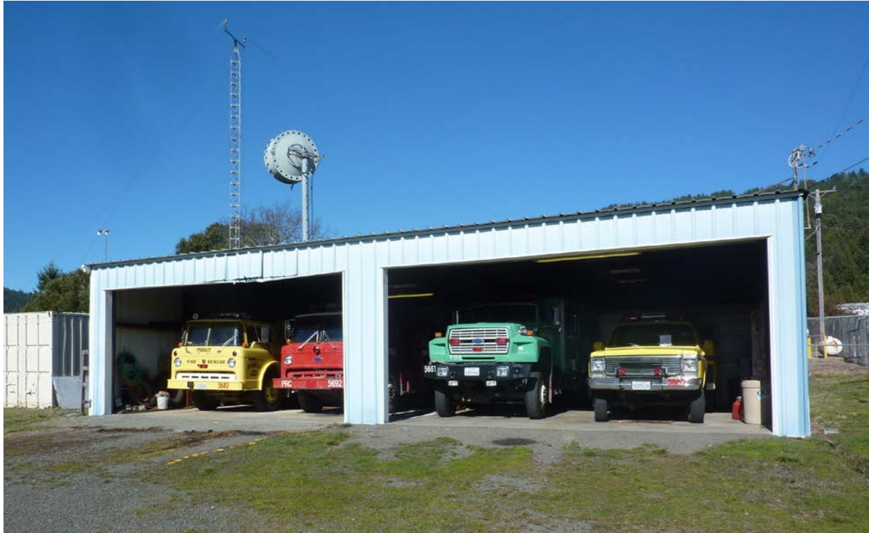
Main Fire Station 80401 Highway 271 Piercy
