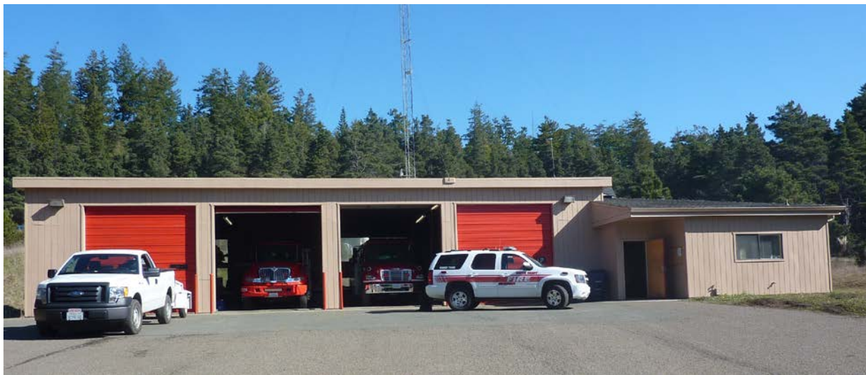
Main Fire Station 39125 Baptist Church Street Gualala
