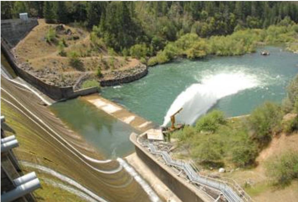
Figure 3-3: Scott Dam at Lake Pillsbury Source: (PVID, 2024)
