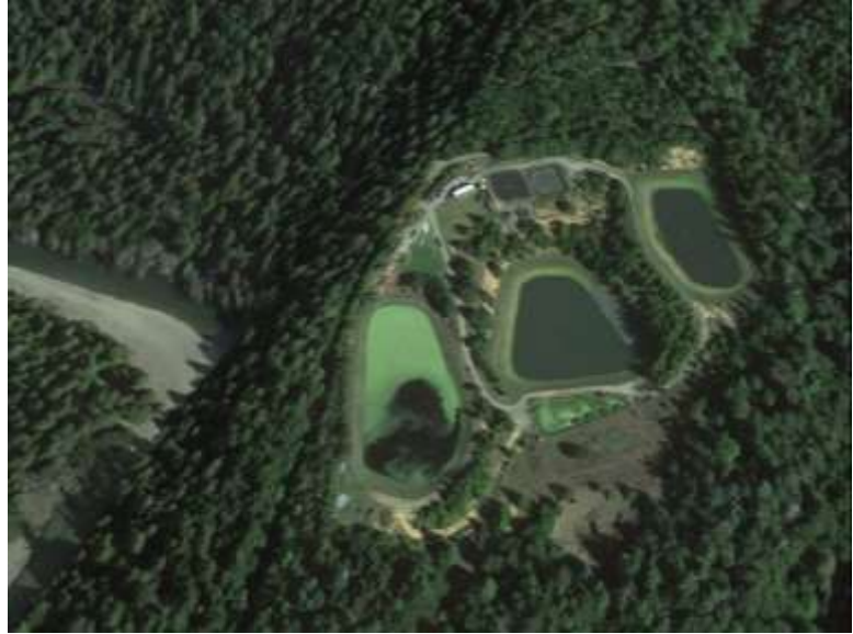
Figure 3-3 Aerial View of GCSD's Treatment Facilities
