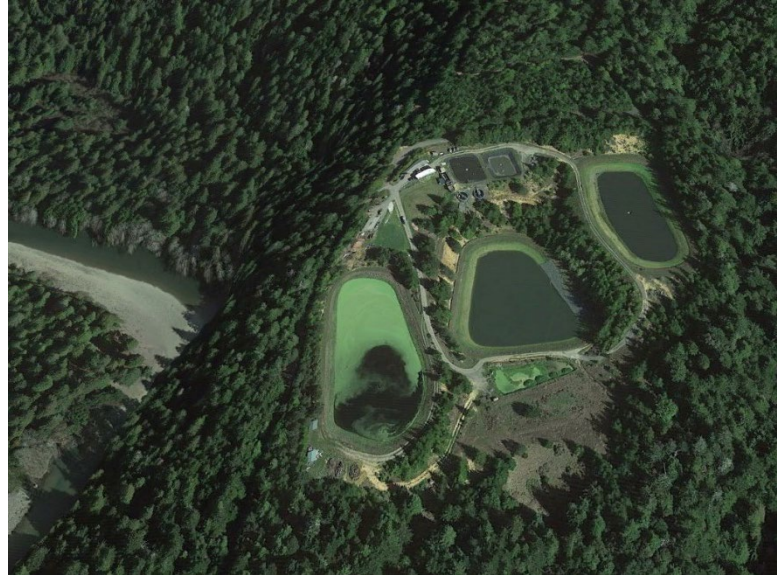
Figure 3-3: Aerial View of GCSD's Treatment Facilities
