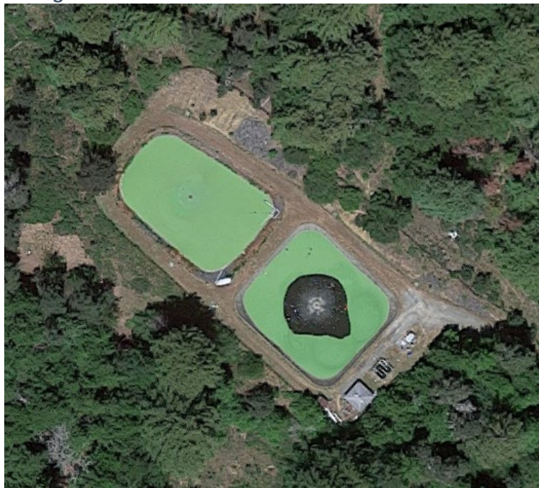
Figure 3-2: Aerial View of Wastewater Treatment Plant
