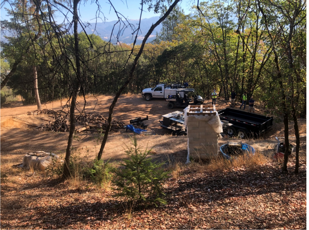
Photo 3. Tank Site #3 (lower)
