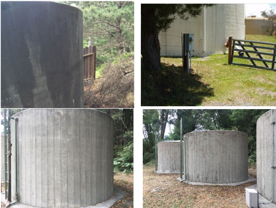
Figure 5. Examples of cast-in-place concrete tanks (North Marin Water District)
