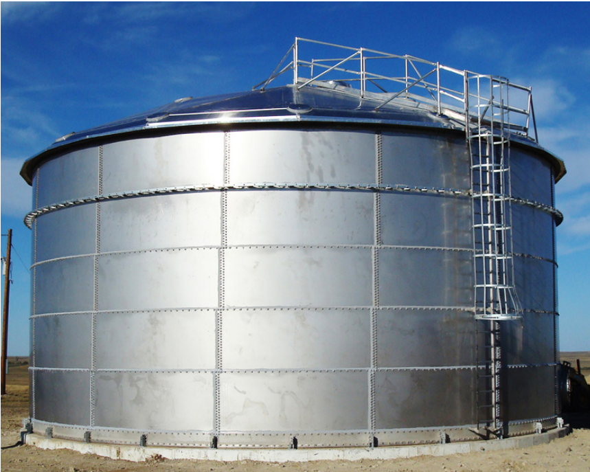
Figure 4. Example of Type 316 stainless steel tanks (American Structures, Inc.)
