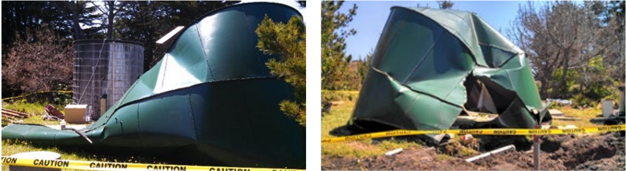
Figure 6. Failed epoxy coated bolted steel water tank (Pacific Reefs Water District)
